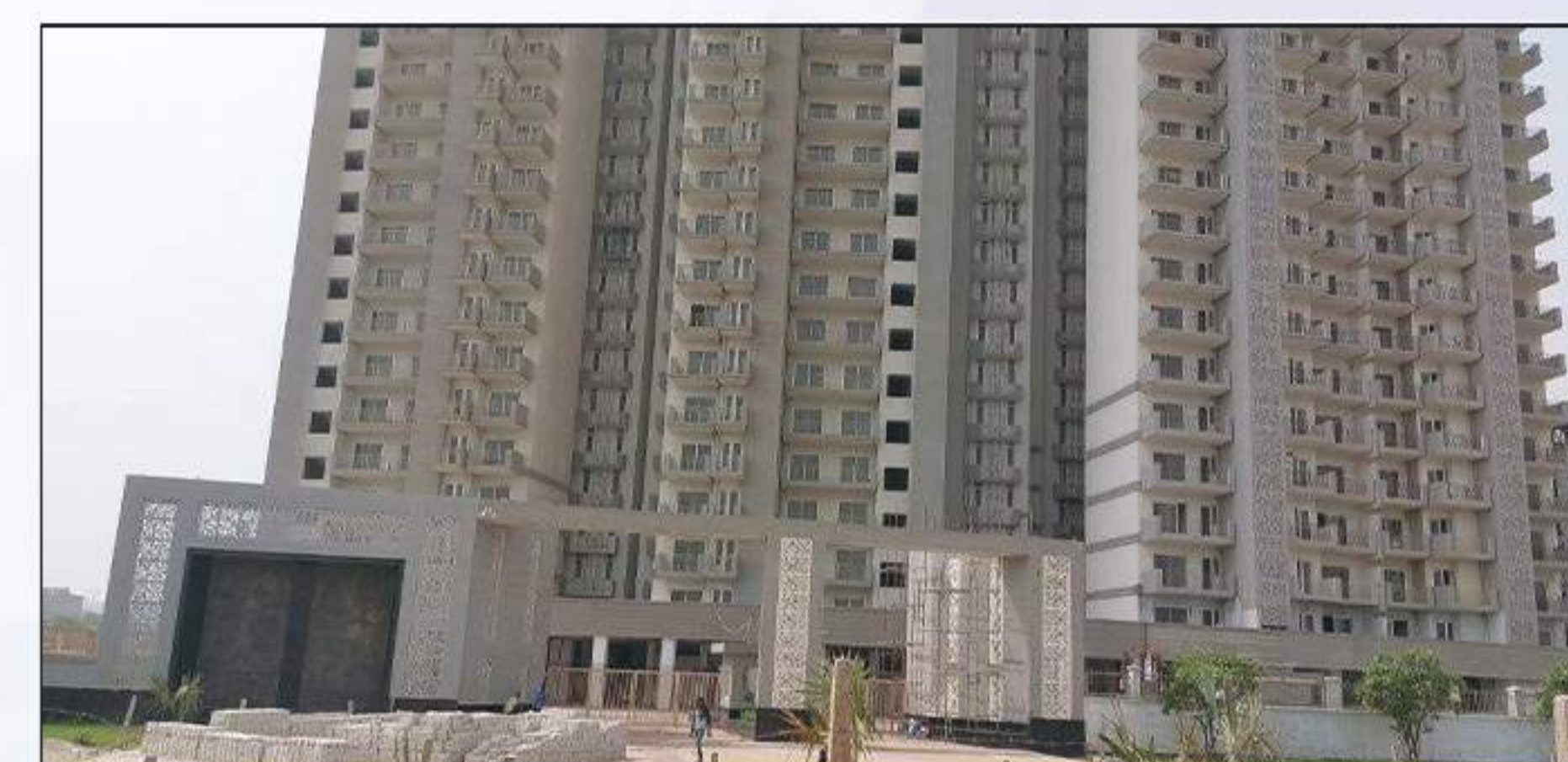
Raksha Towers, Micasa, Sec68, Gurgaon
